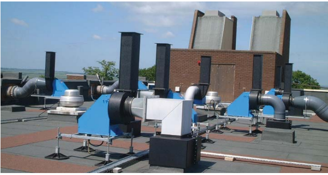
Big Foot installed to support extractor system
